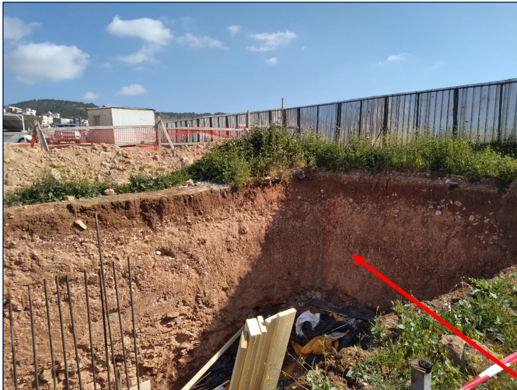
FIGURE #07& 08: Possibility of soil sliding, it is recommended to protect the area.
