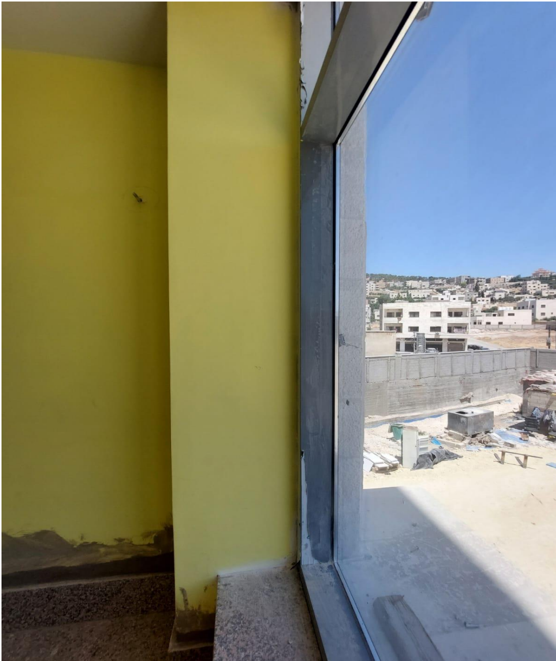
Rectifying the fixation of aluminum Curtain wall
