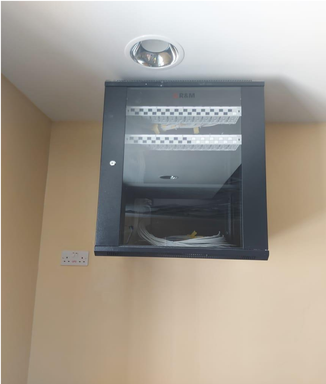
Re-installing of Data System cabinet without causing damages
