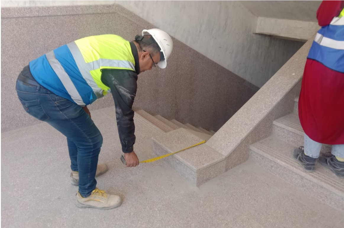
Dissimilarity at the main staircase
