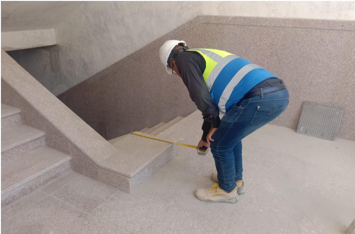
Dissimilarity at the main staircase
