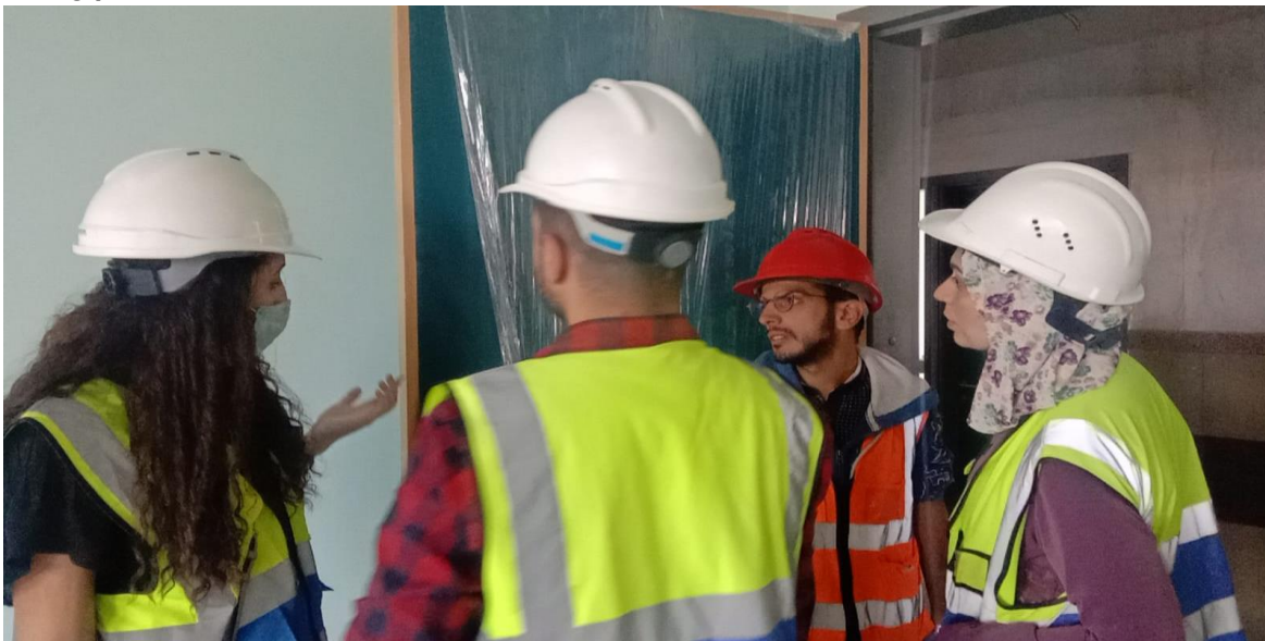
Unprotected wooden doors
