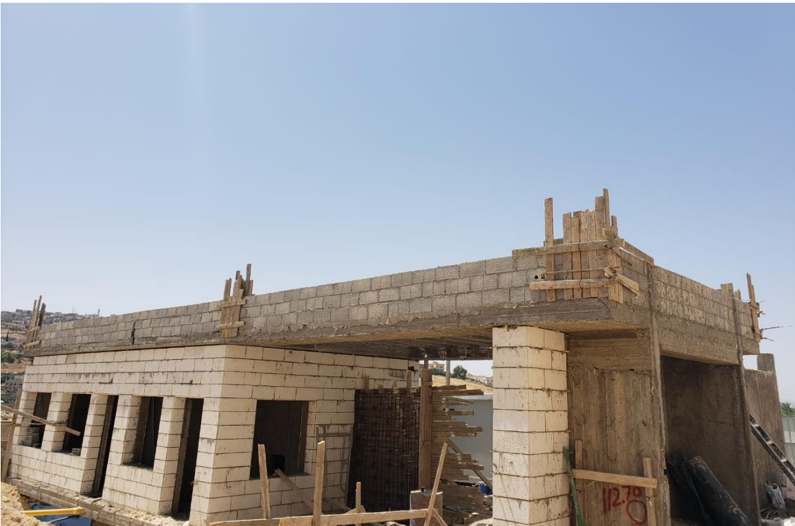
Creating stiffener columns in the parapet
