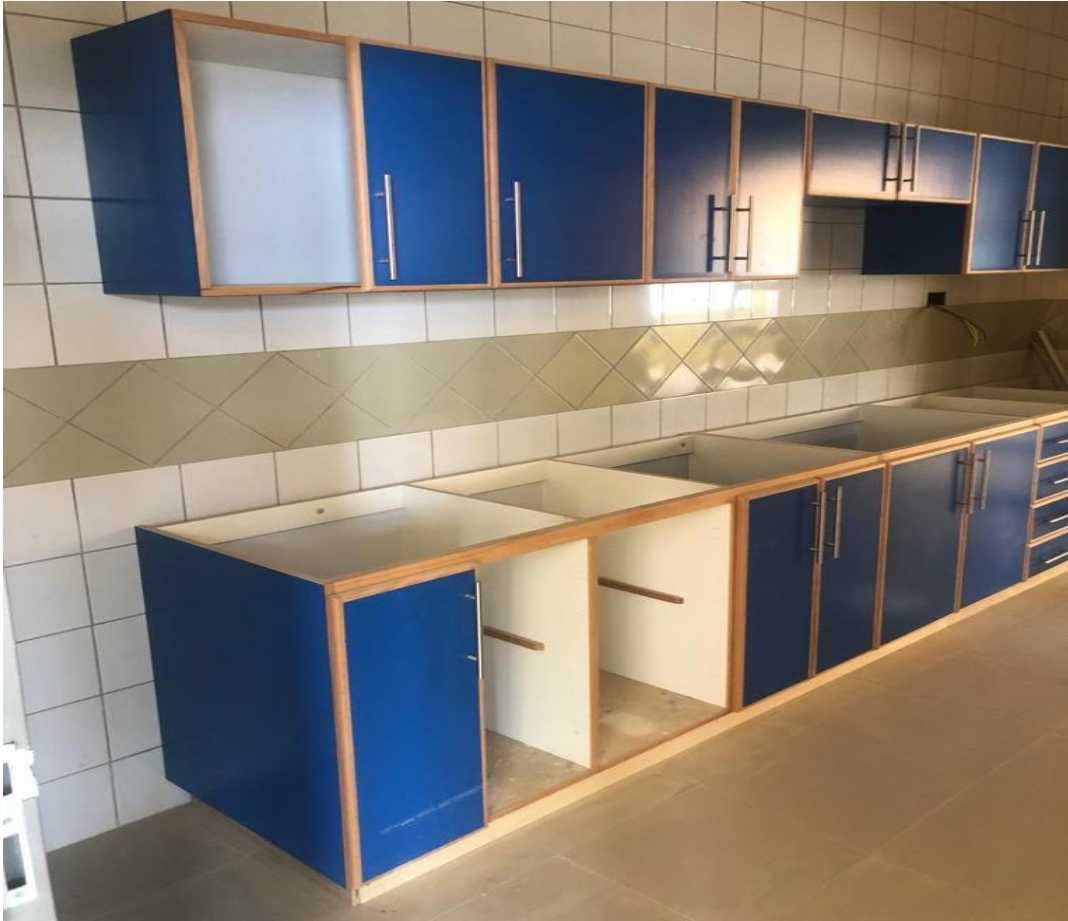
Removing defected parts for rectification
