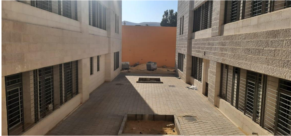
Interlock tiling at the Core area between Zones A and B
