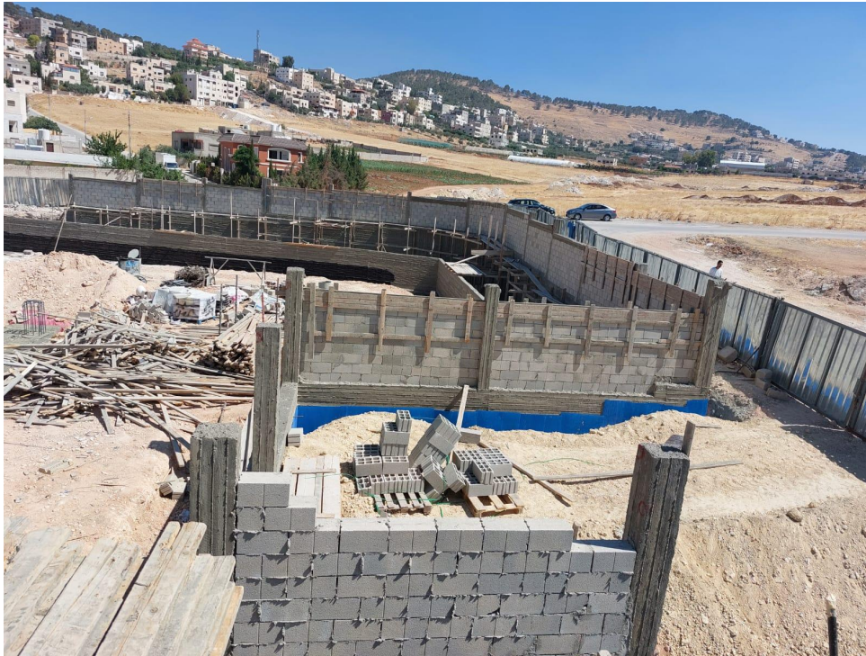
Blockwork for the boundary walls no.01 and 07
