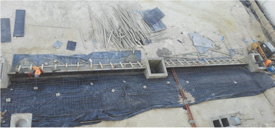
Formwork and steel reinforcement for the amphitheatre
