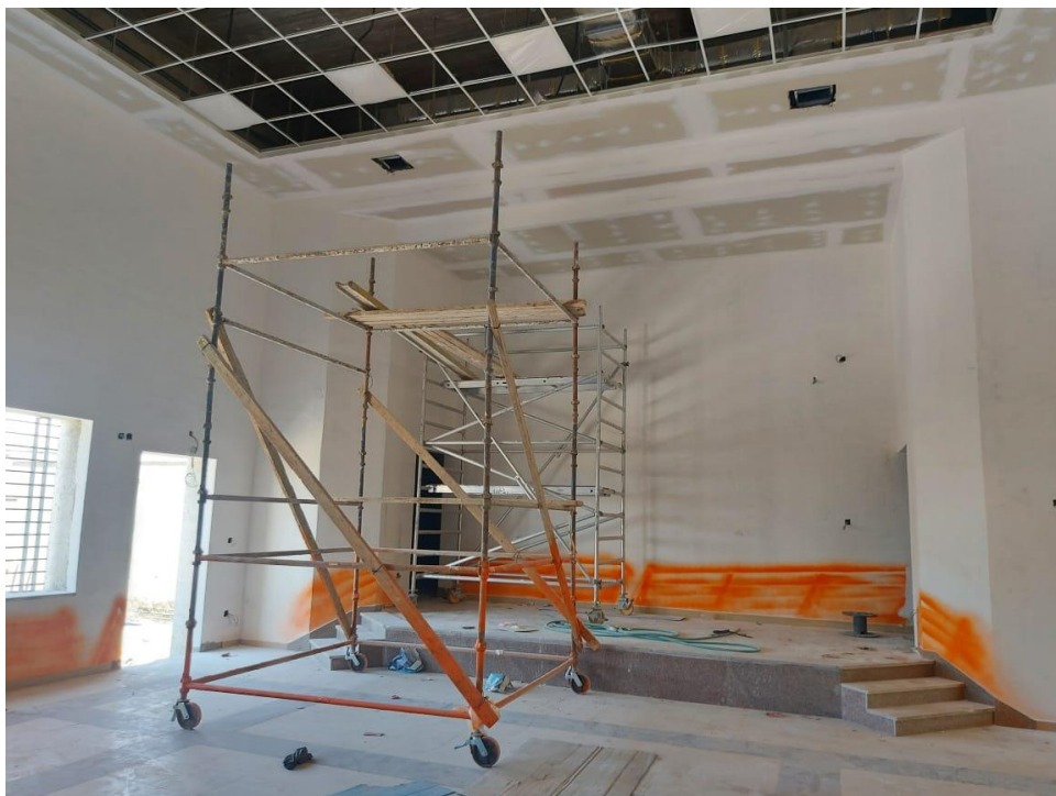
Suspended ceiling and painting works at the multi-purpose hall
