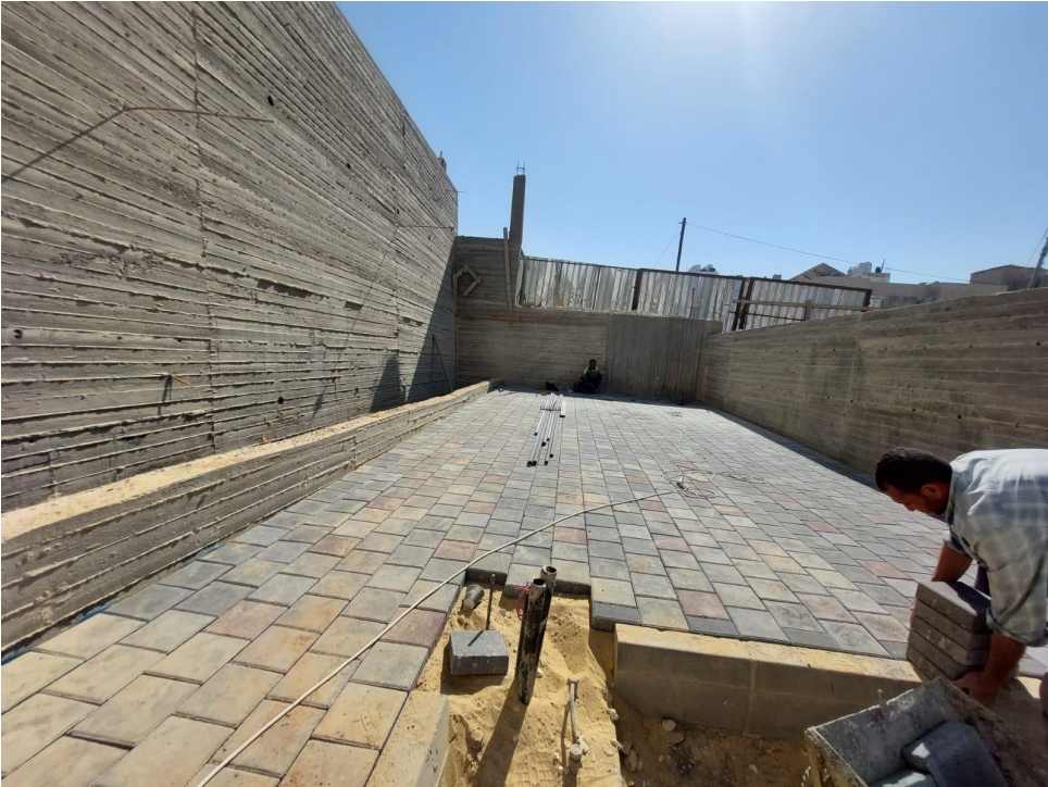
Interlock tiling at the south- eastern side of the building
