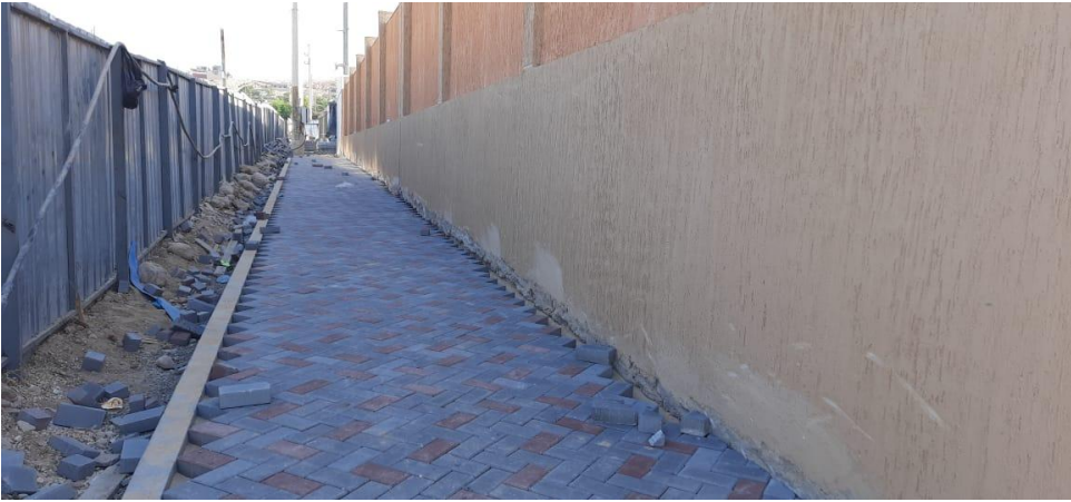
Interlock tiling for the sidewalks
