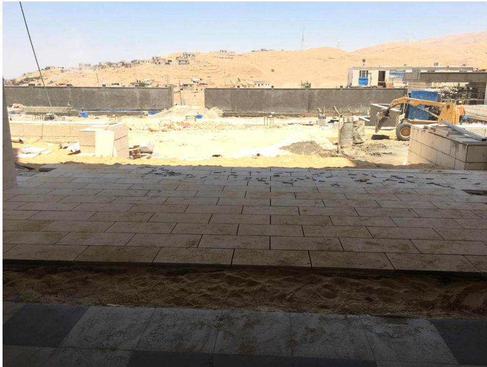
Stone tiling for the main entrance at Zone B
