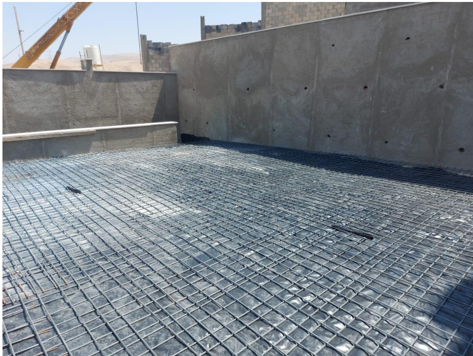
Steel reinforcement for the multi-purpose hall terrace
