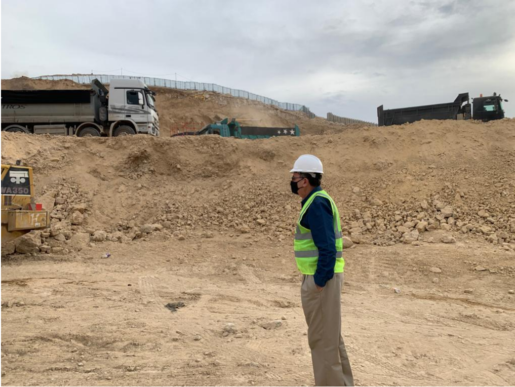
Engineer Wahib observing the progress of the excavation works
