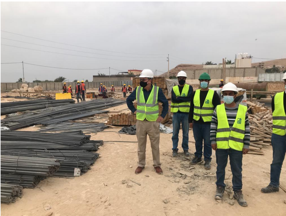
Observing work progress at the site
