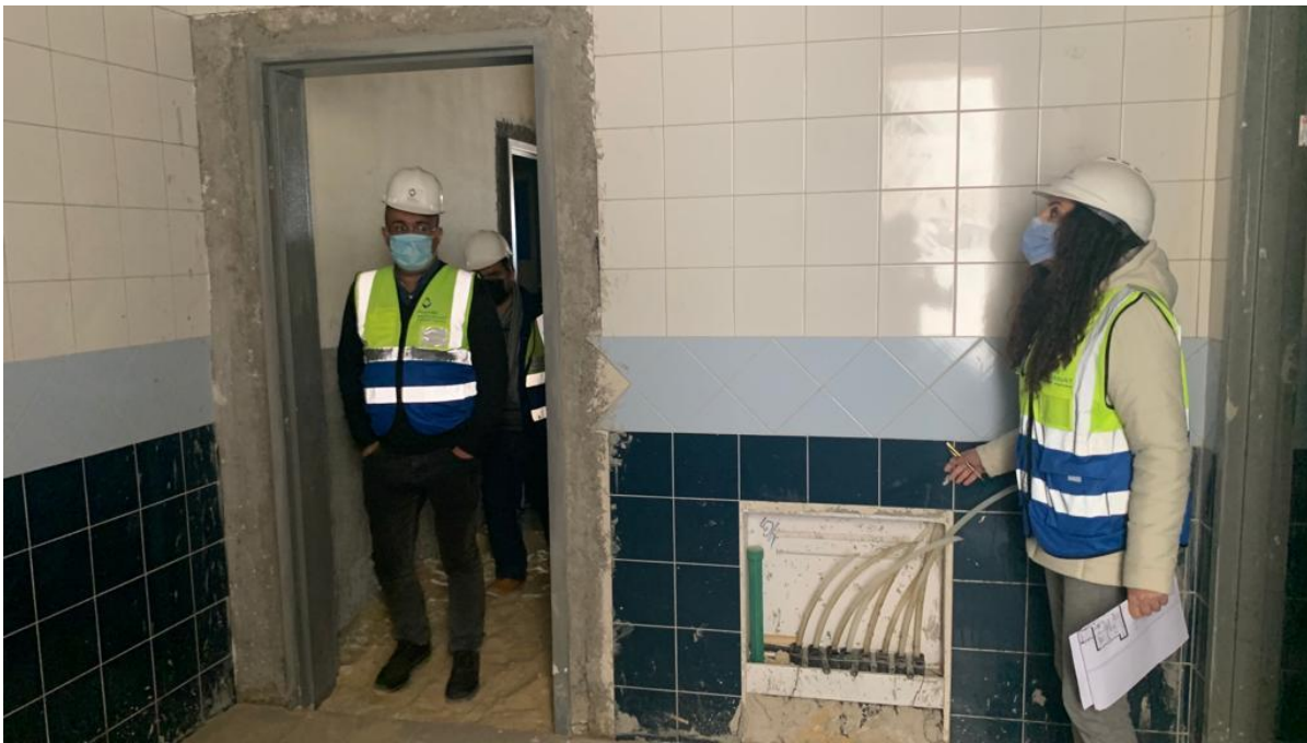
Inspecting the wall tiling work at the wet areas
