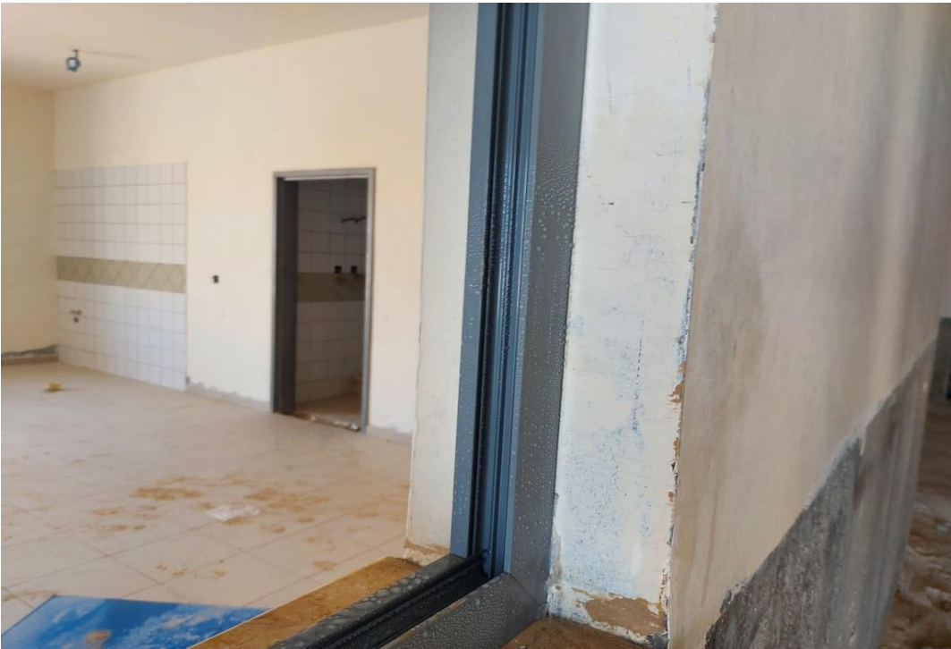
Unfinished window jambs
