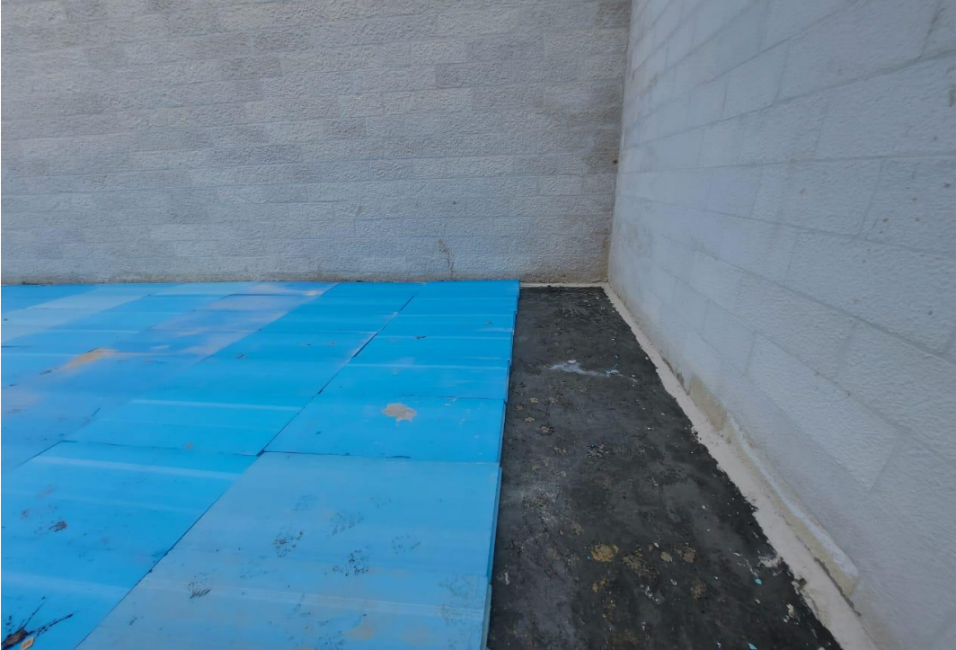
Waterproofing for the roof of multi-purpose hall
