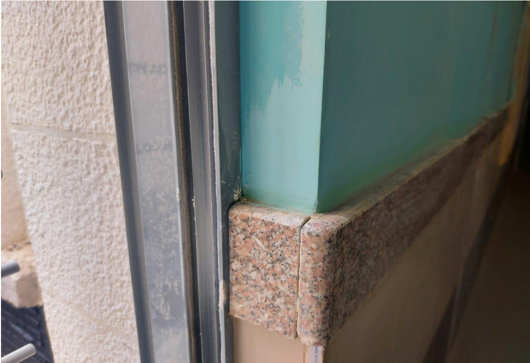
Rectified granite coping
