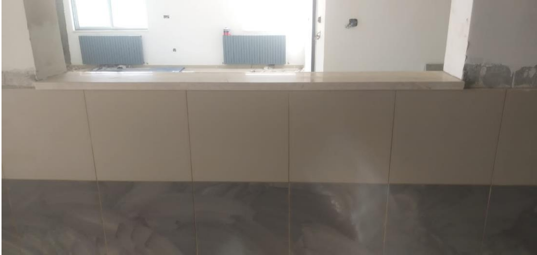
Rectified window sill
