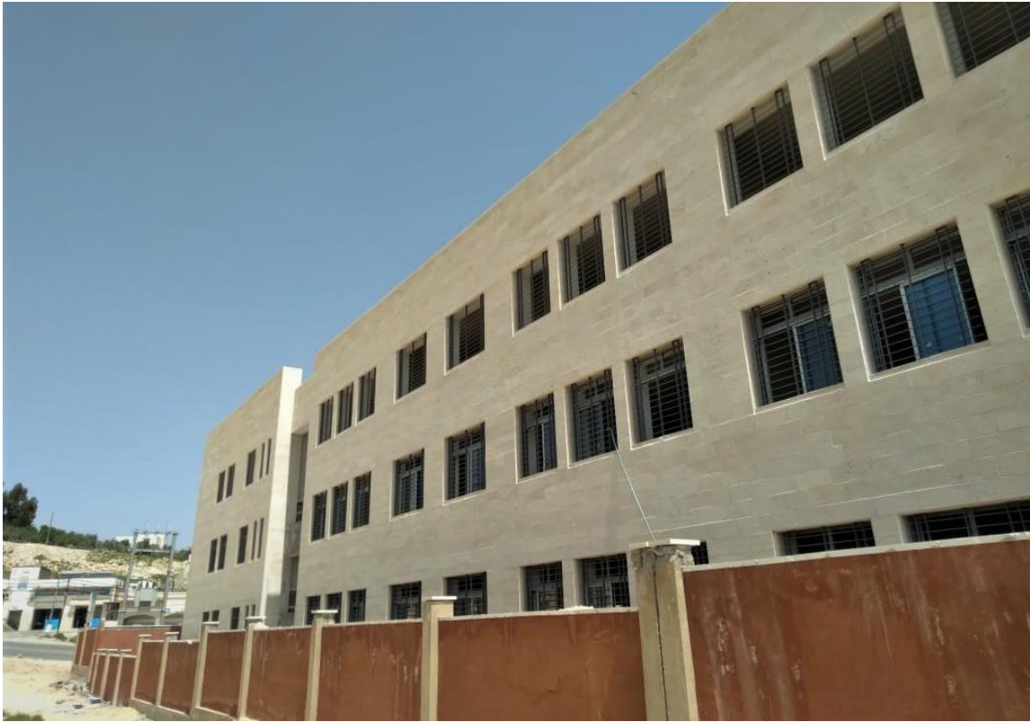
General view of the project
