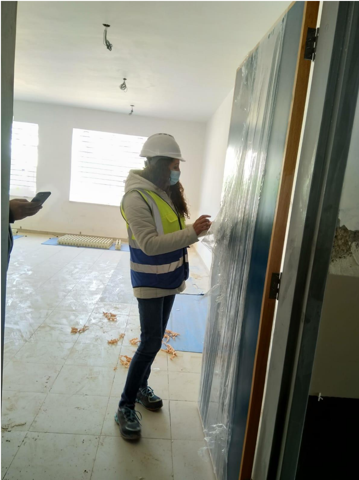
The Supervision team inspected the installed door samples (figure:07 & 08)
