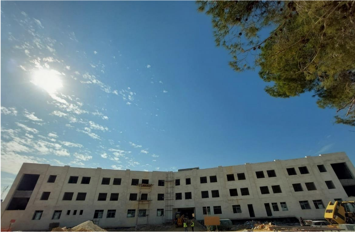
General view of the project site (figure:01, 02, 03)
