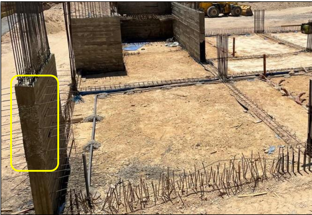
Figure 9: Concrete Segregation
