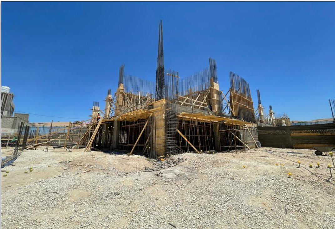
Figure 1&2 : Construction site and main ongoing activities
