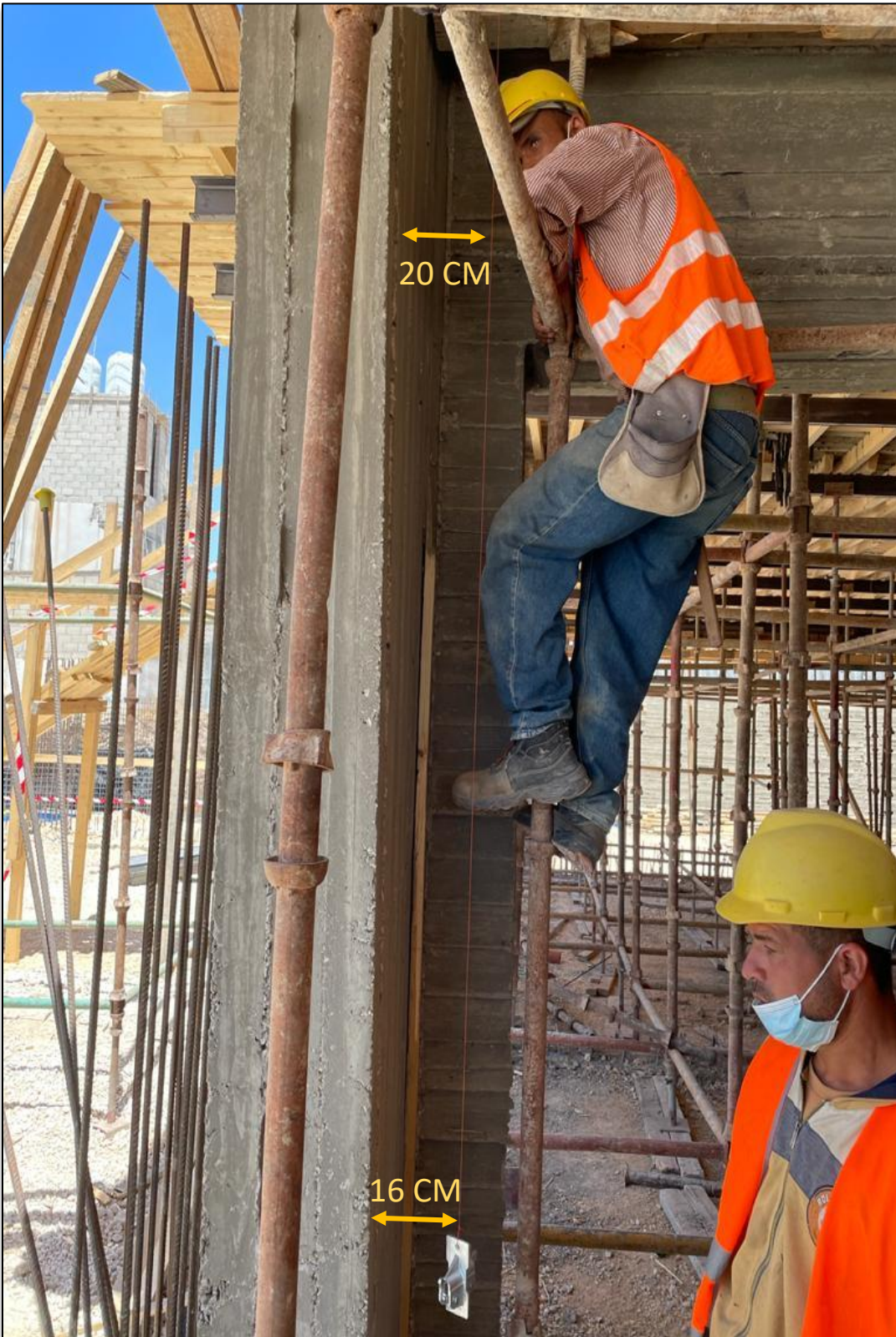
Figure 7: Measuring Column plumbness
