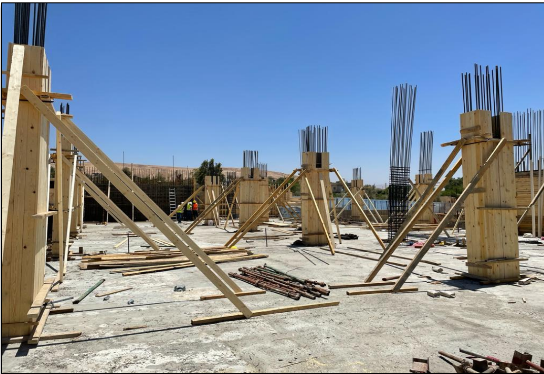
Figure 6: Preparing Columns of First floor
