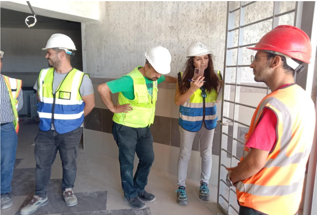
Door part does not comply with architectural details
