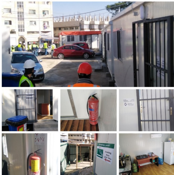
Figure #4: The site office area was inspected and appeared in a compliant condition. Adequate site office trailers with secured doors, safety signs, waste containers, smoking area, and temporary kitchen available. Plus, fire extinguishers provided and assembly point identified. Photo credit: Odai Tawalbeh, 12/1/2020
