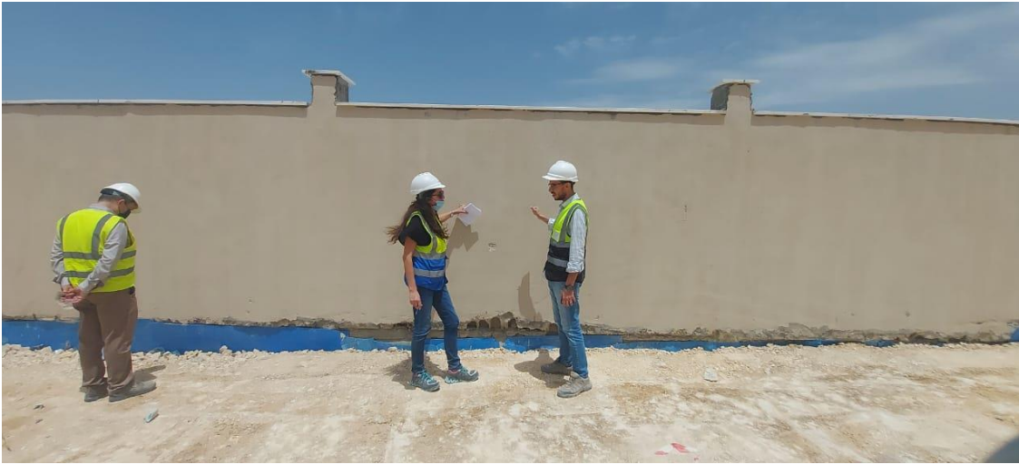
Inspecting the external colored plastering sample for boundary walls
