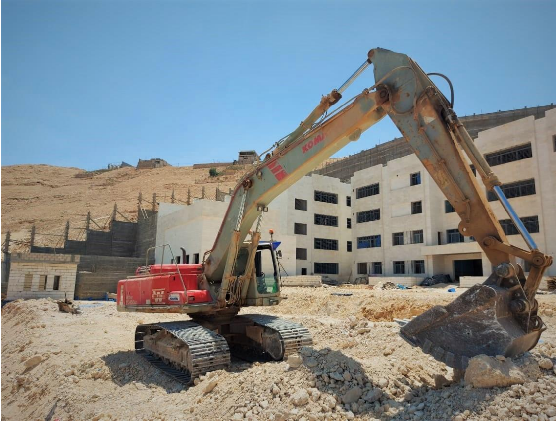
General view of the project site (Figure: 01, 02, 03 & 04)
