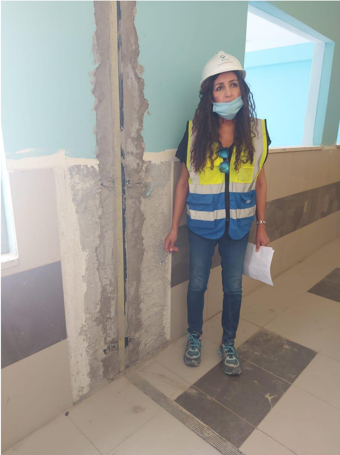
The team inspected the executed expansion joints at the corridors
