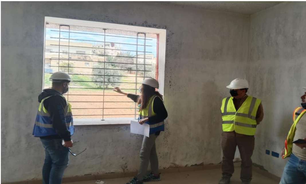
Corrosion appears on the steel protection screens
