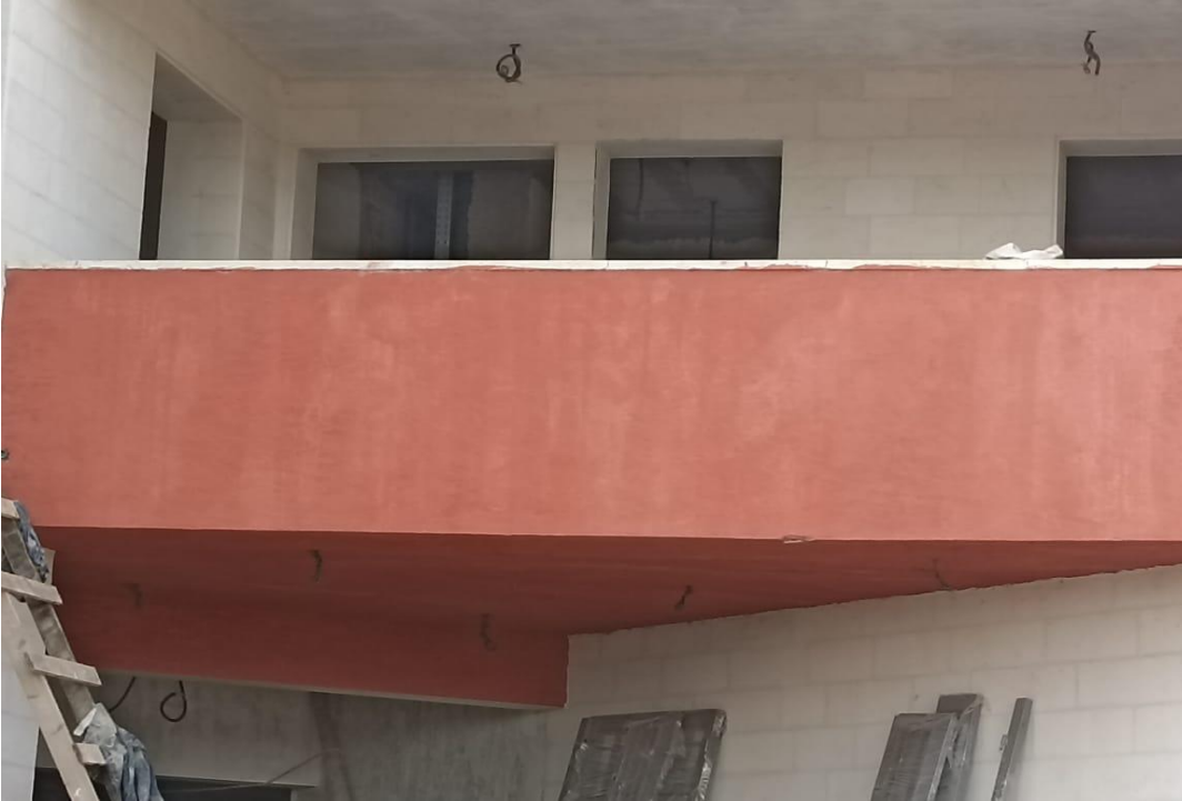
Rectified external plastering
