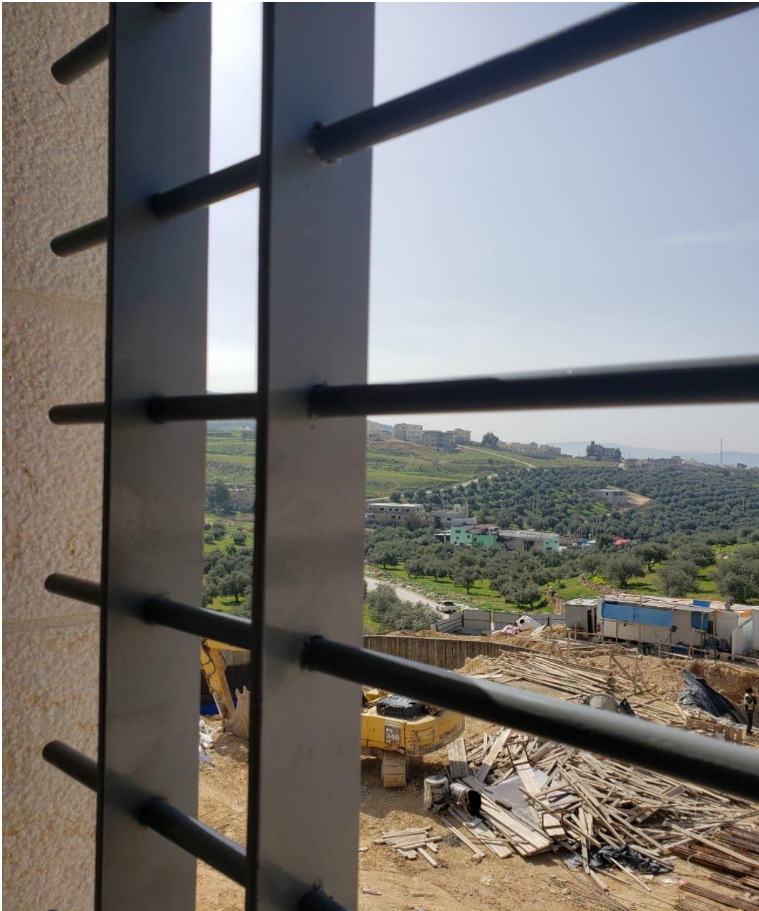
Rectified paint for the steel protection screens
