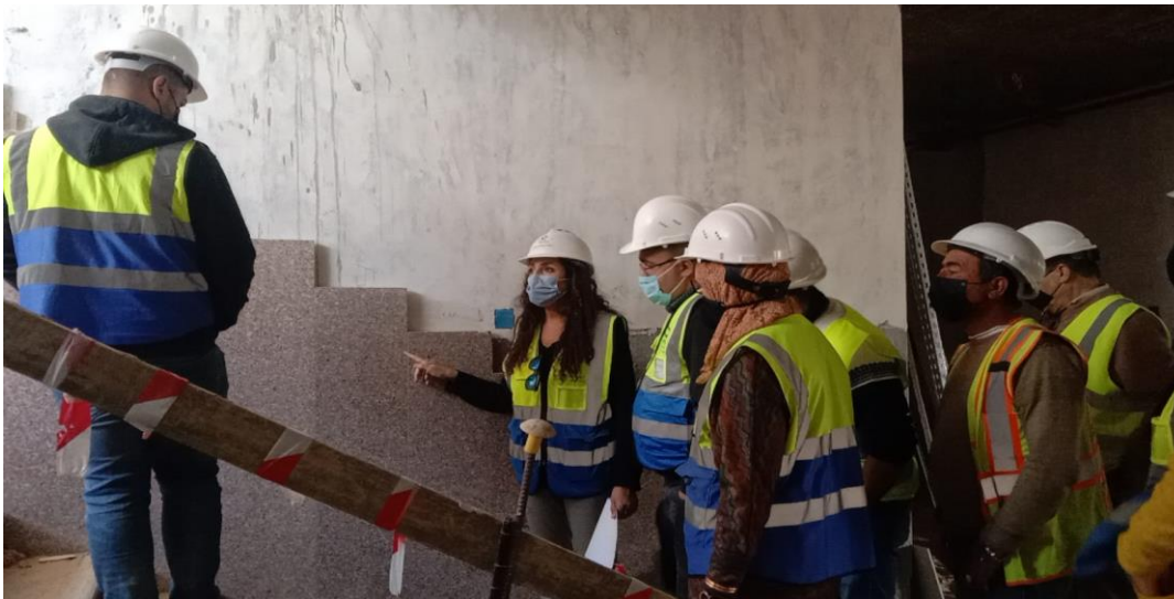
Defects in the granite cladding for staircase walls
