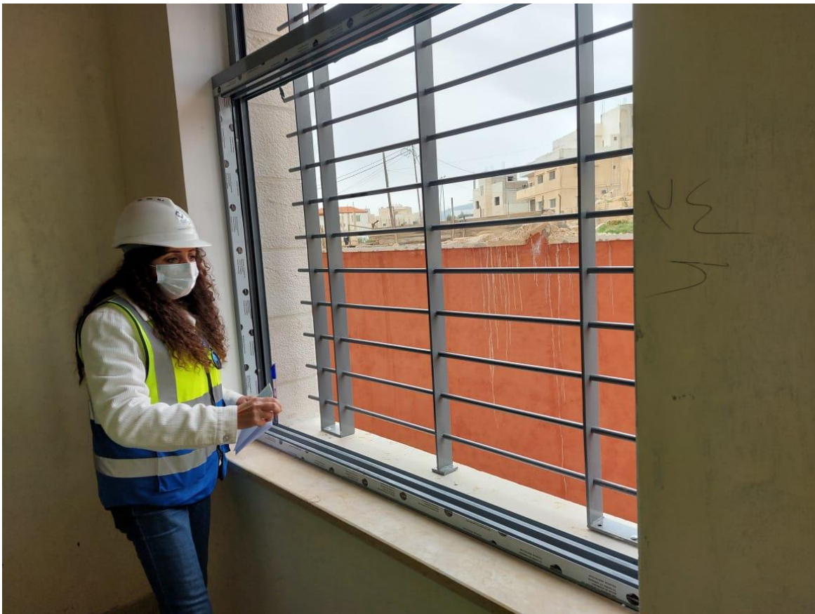
The team inspected the fixation of aluminum window frames for windows
