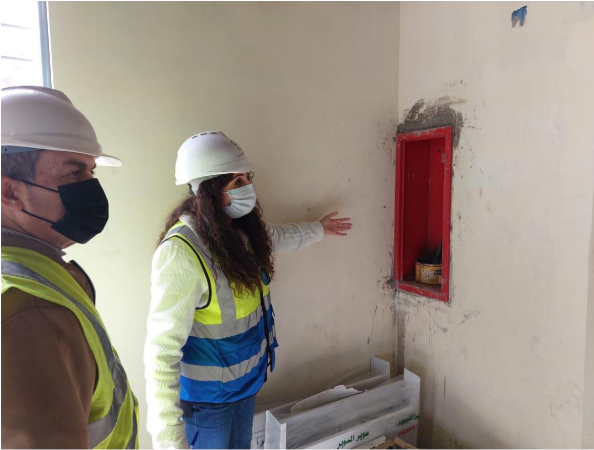
Inspecting fire extinguisher installation at the multi-purpose hall
