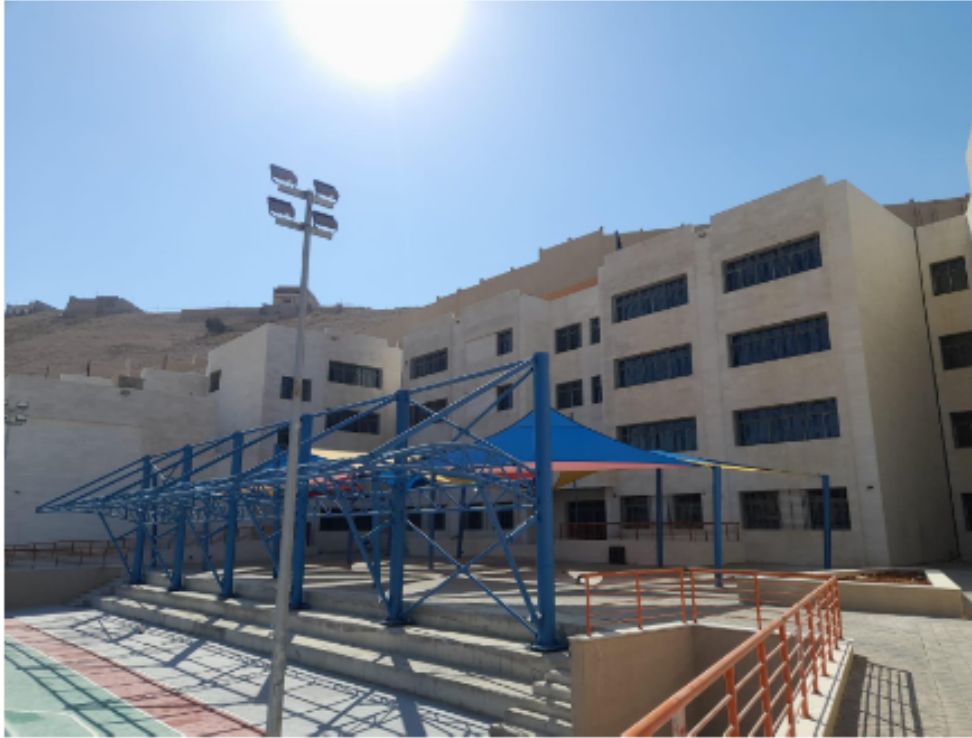
General view of the project site (figure: 01 & 02)
