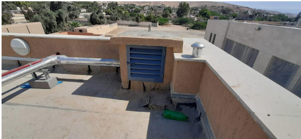
Installing window louvres for the shafts at the roof
