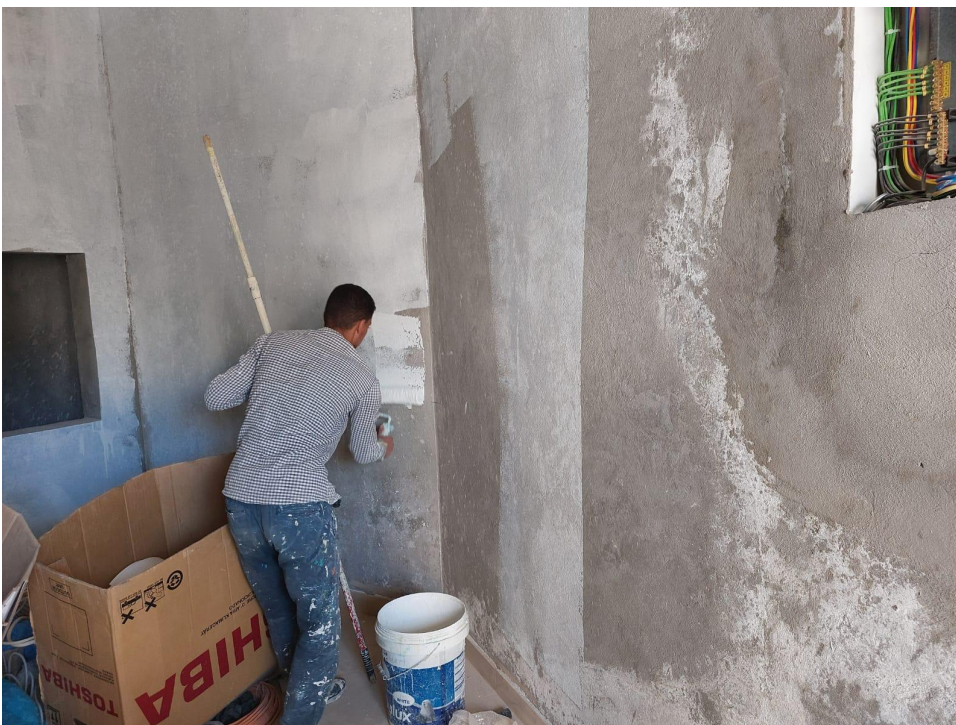
Finishing electrical and plastering works at the main electrical room
