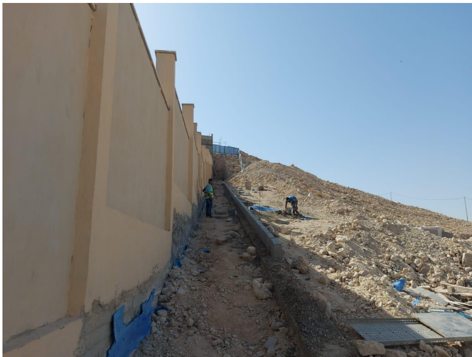
Starting works at the sidewalks next to the KG classrooms
