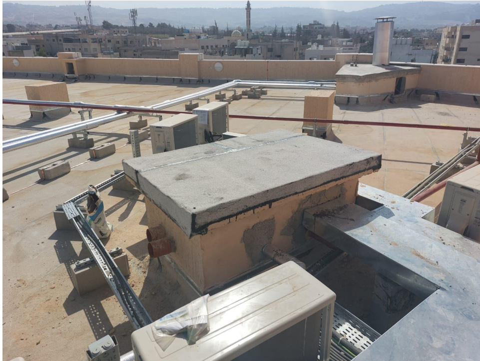
Insulation works for shafts' tops at the roof
