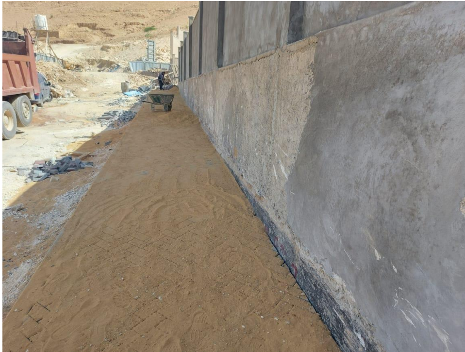
Finishing works at the sidewalks
