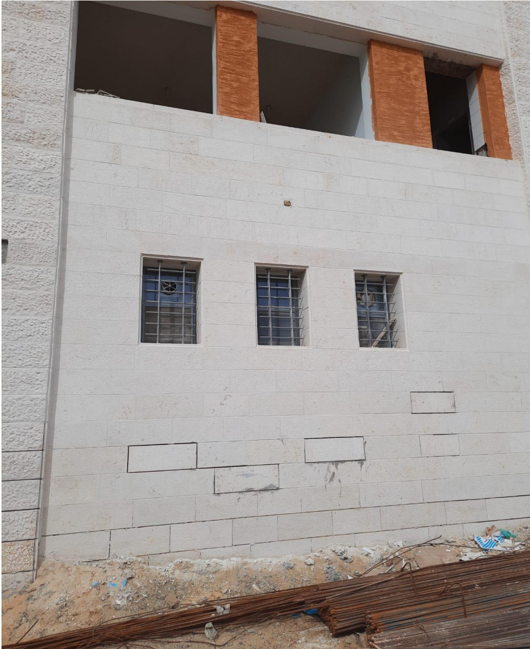
Replacing defected stones and removal of debris
