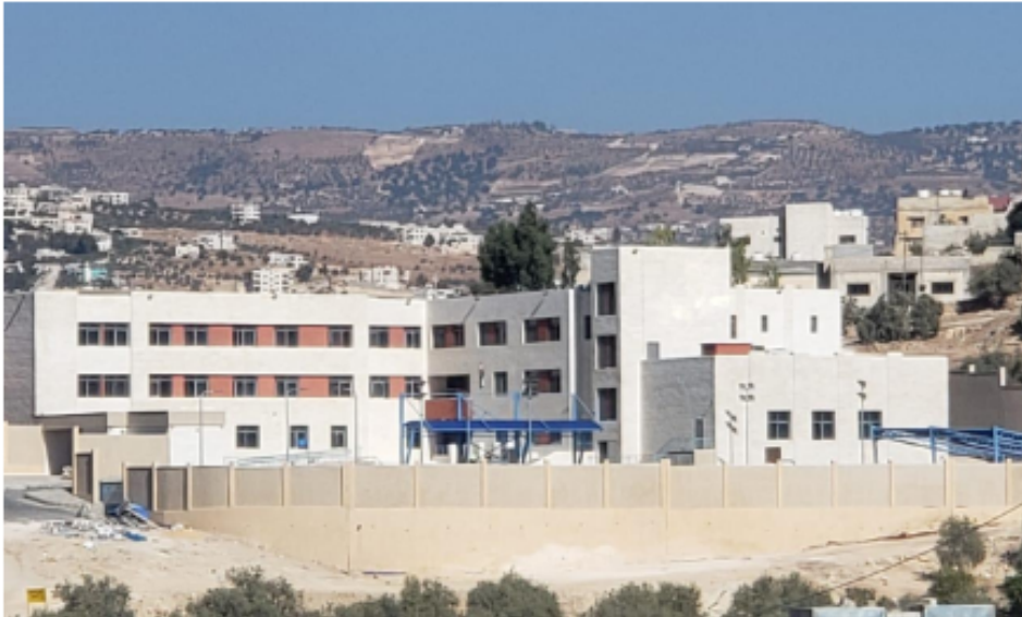
General view of the project site
