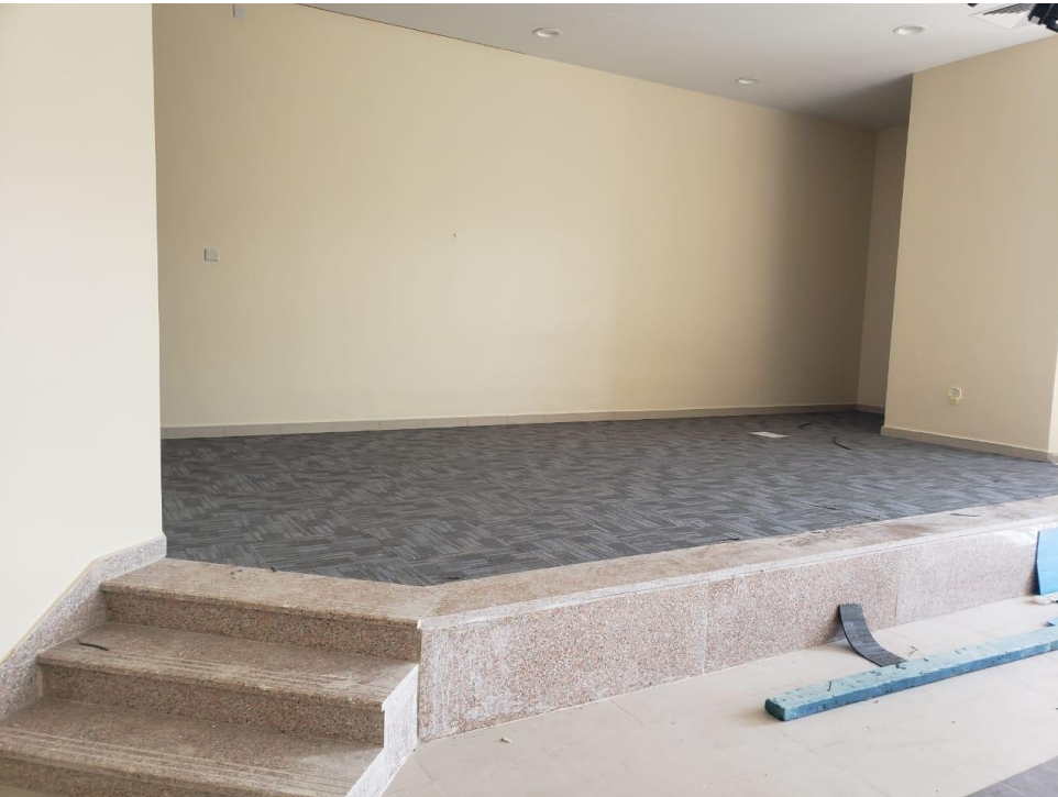
Installing the carpet at the multi-purpose hall
