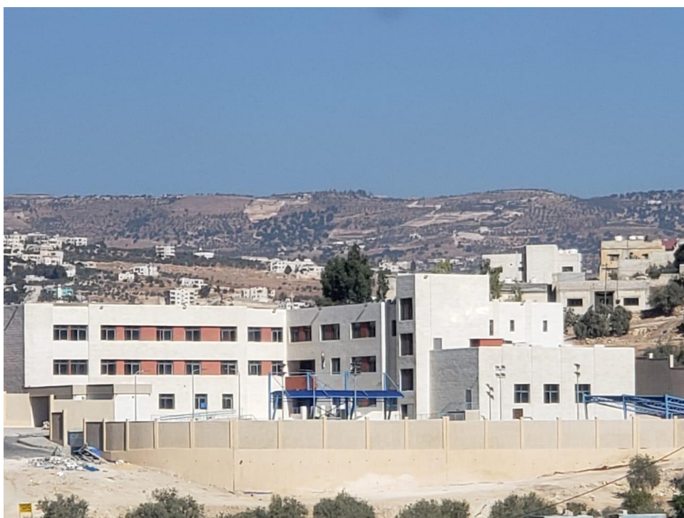
General view of the project site
