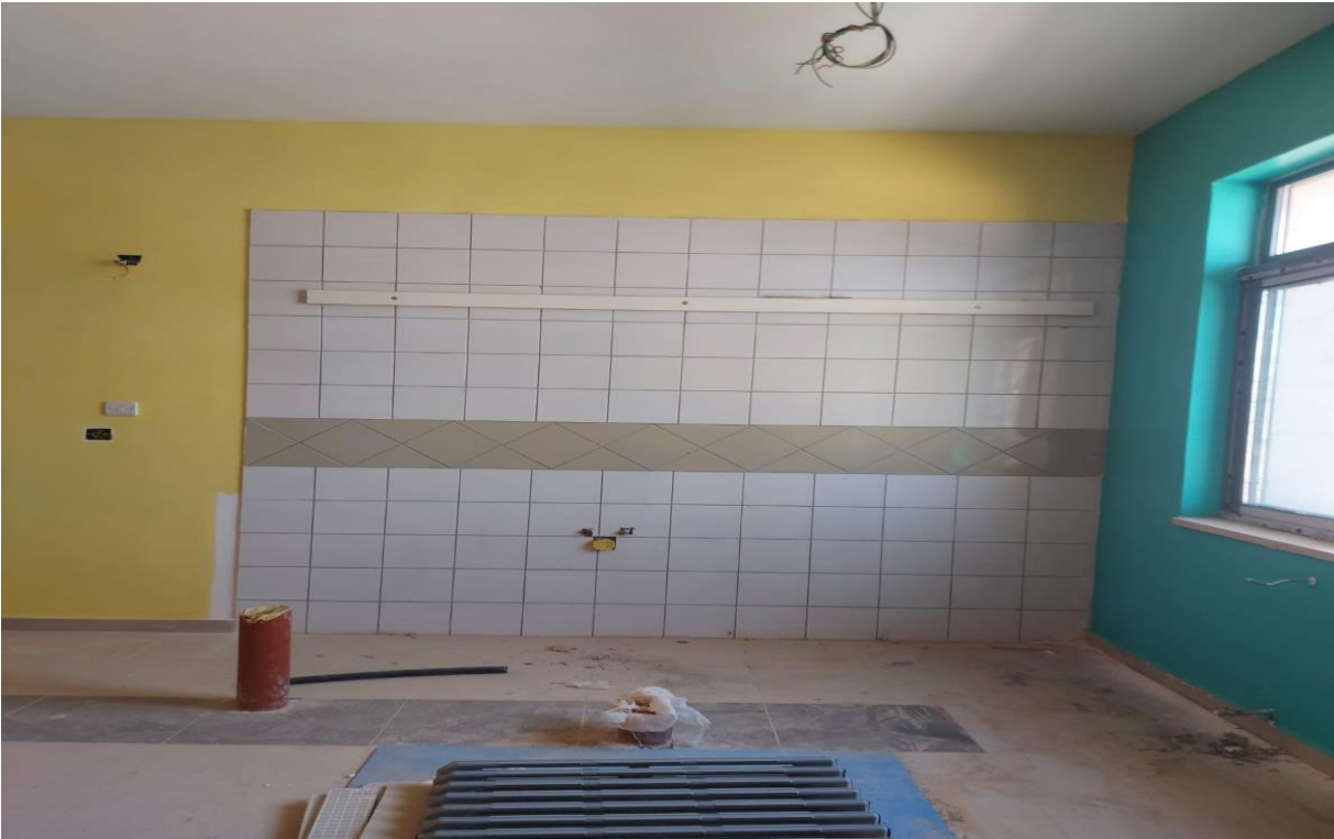
Removal of defected cabinets
