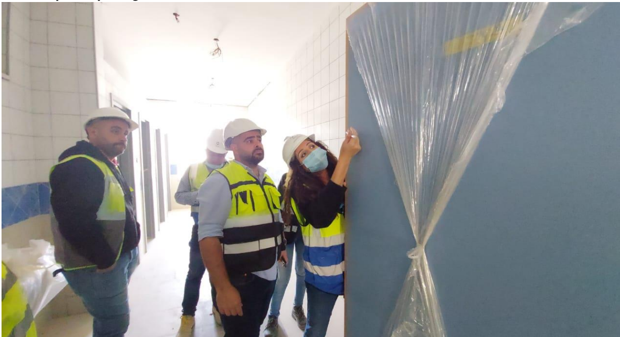
Unprotected door leafs
