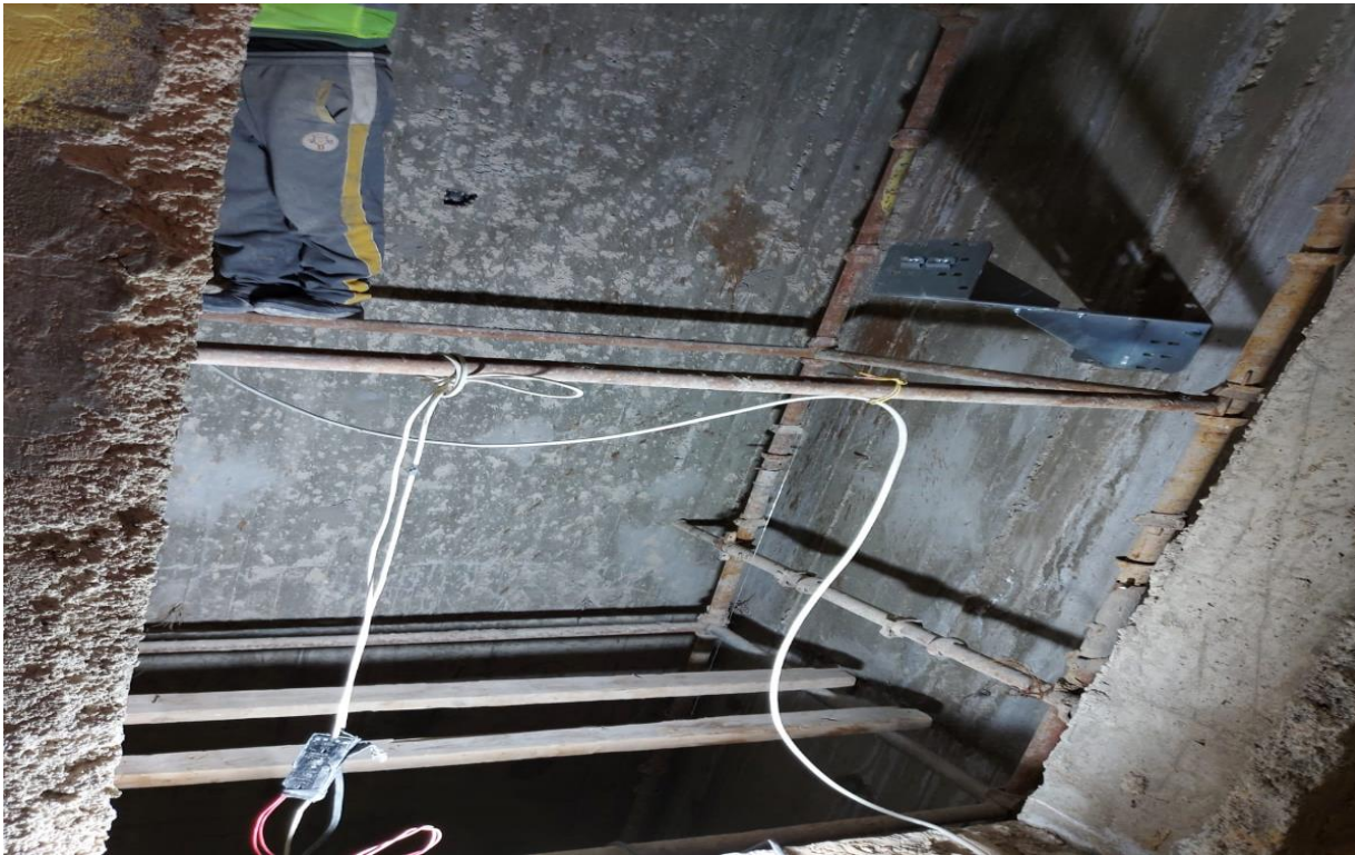
Installation of elevator
