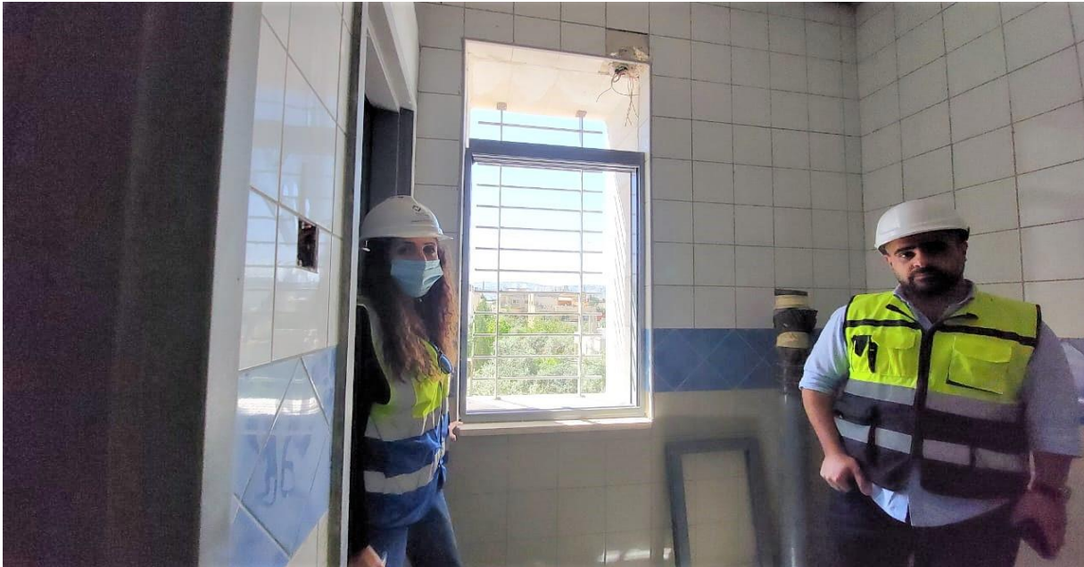
Wrong dimension of aluminum sections
