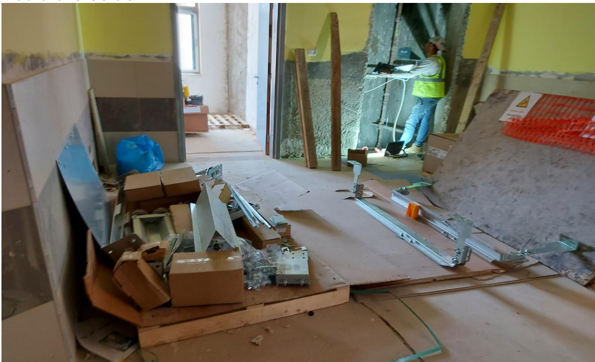
Installation of elevator
