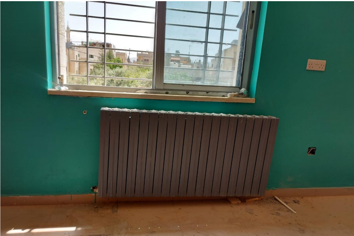
Desmantling of radiator to allow opening to the cabinet
