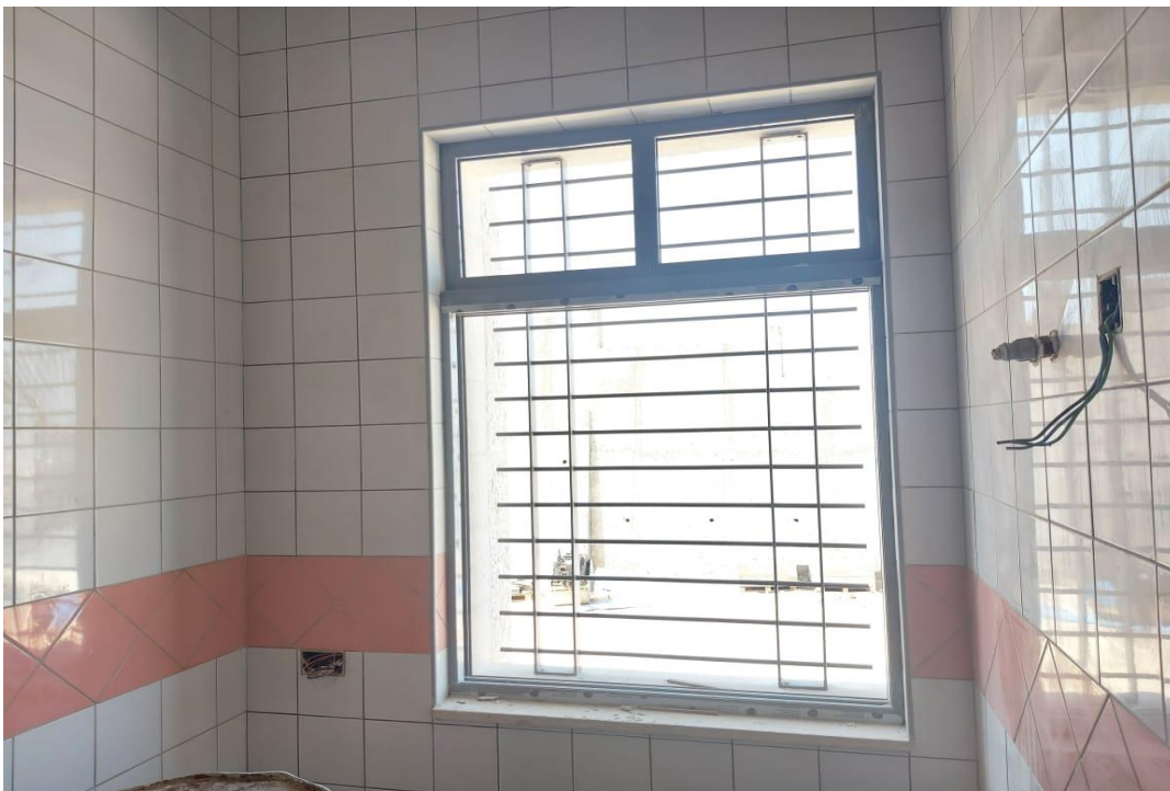
Re-tiling of ceramic wall tiles
