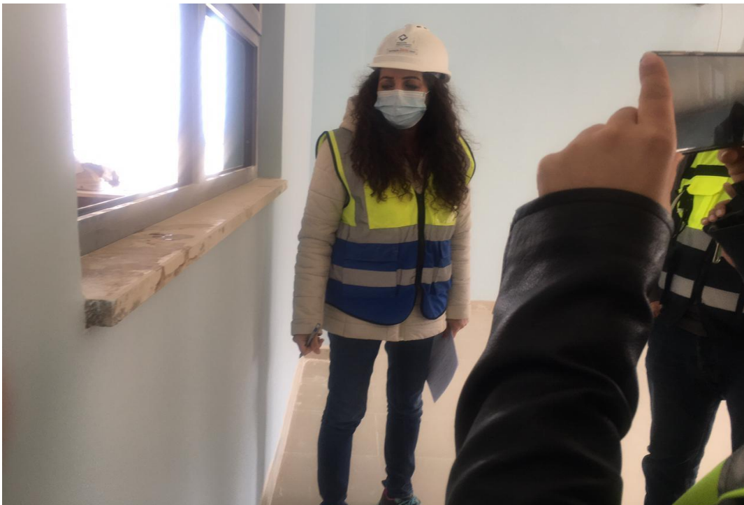
Broken window sill
