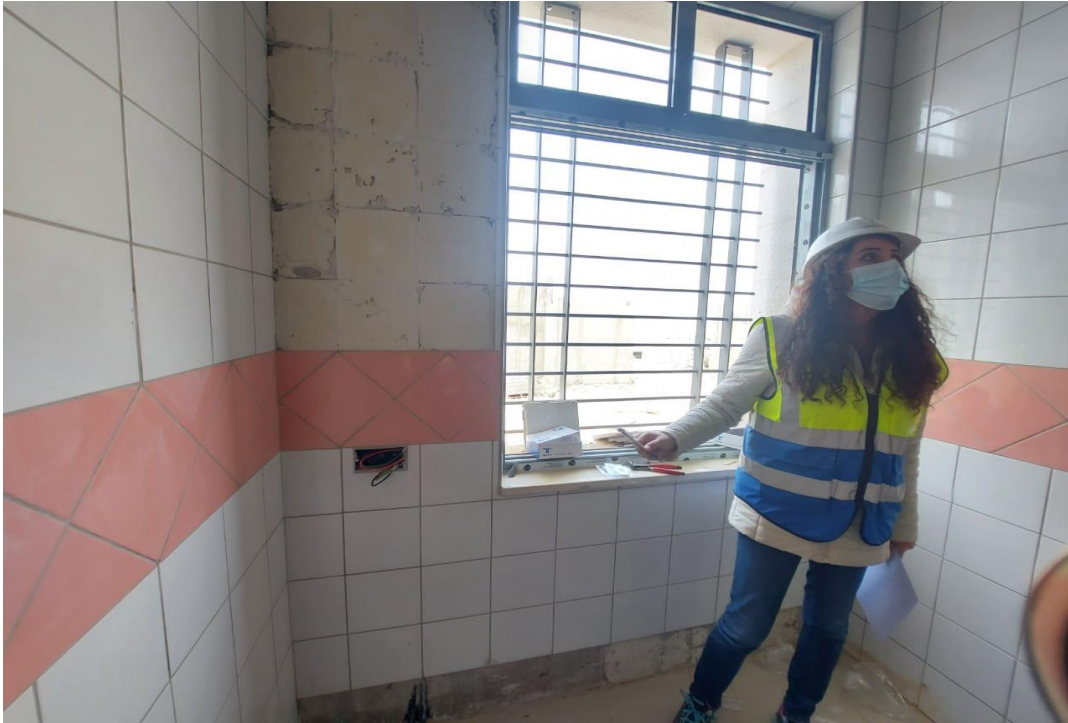
Removal of defected installed tiles
