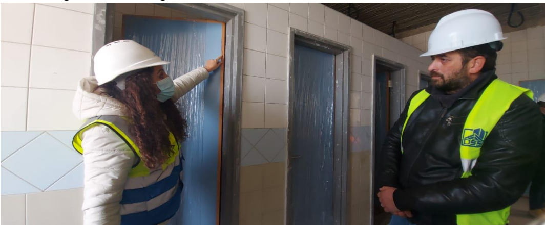
Defects in beech wood frame
