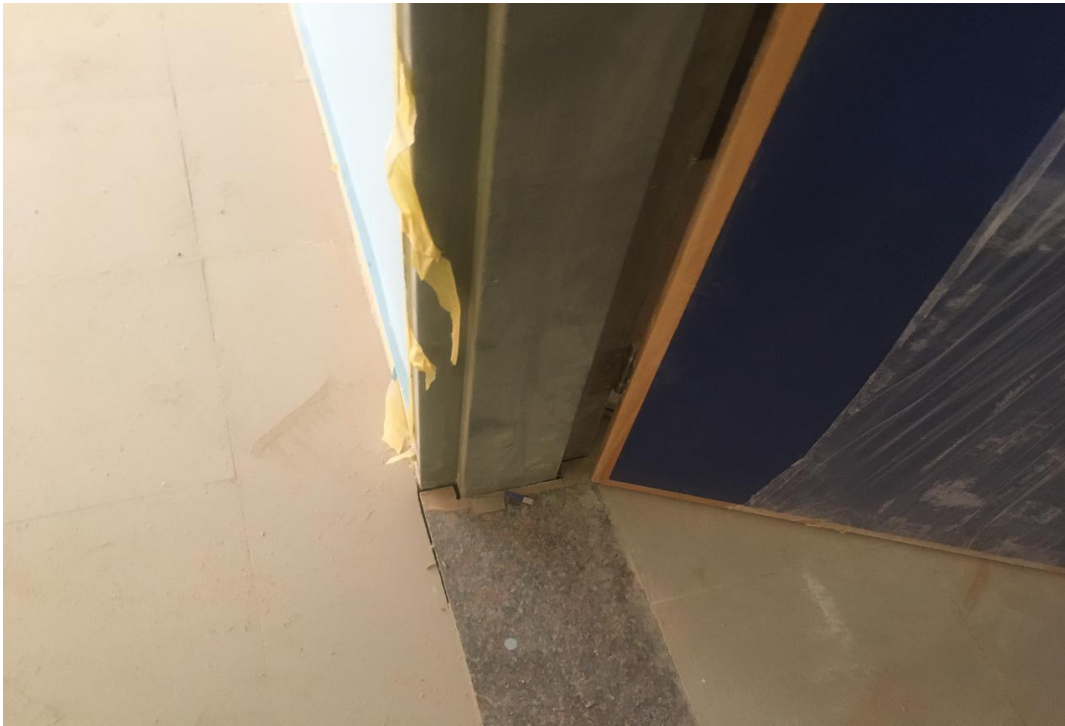
Unlevelled threshold
